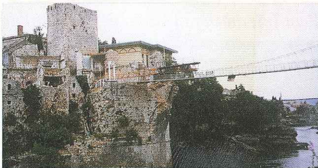
The British Army constructed this temporary bridge to replace the historic Bridge of Mostar (now rebuilt)
